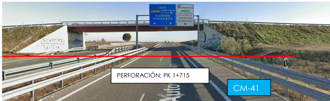
Figura 1 Vista PHD Carretera CM-41
